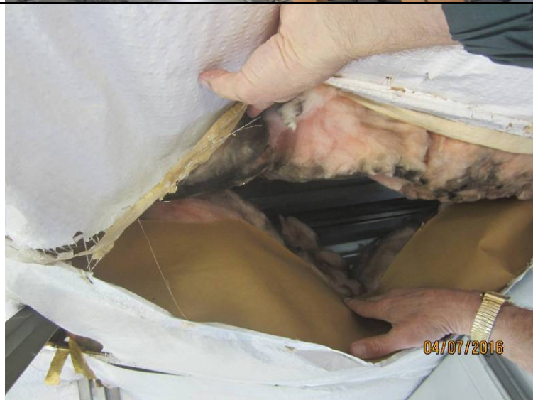
Photograph 24: Fiberglass batt insulation exposed.
