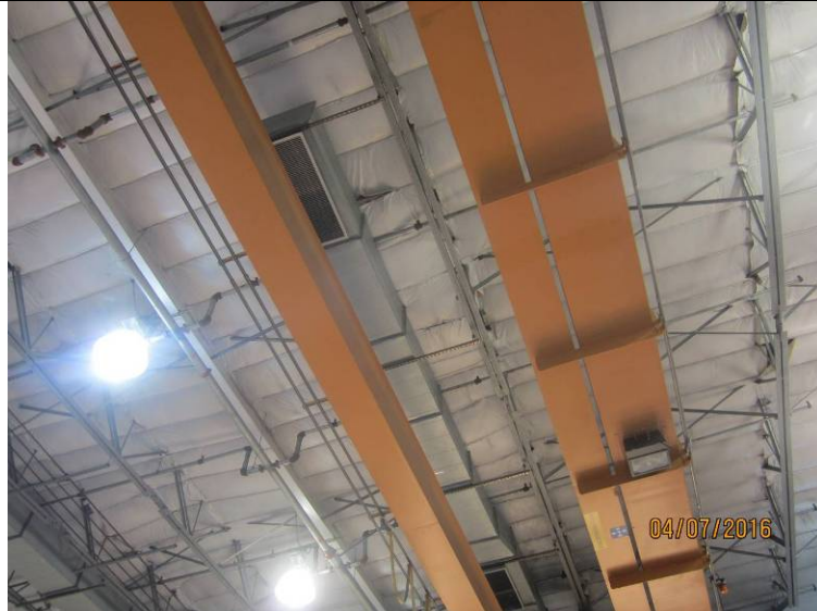
Photograph 23: Looking up at the underside of the insulation and vapor barrier form within the Maintenance Shop.
