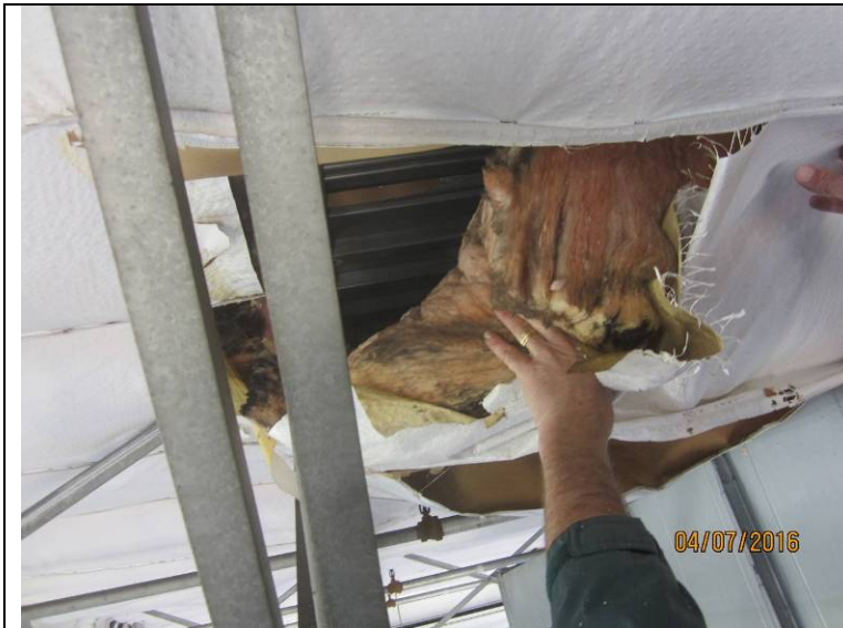
Photograph 25: Additional location of exposed fiberglass insulation with signs of dirt accumulation.
