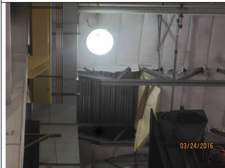
Photograph 3: A location of missing insulation exposing the underside of the metal roof deck.
