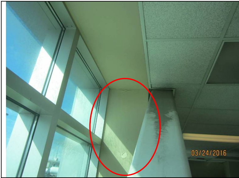
Photograph 45: Area below the sill track shown in Photograph 43 showing signs of water entry.
