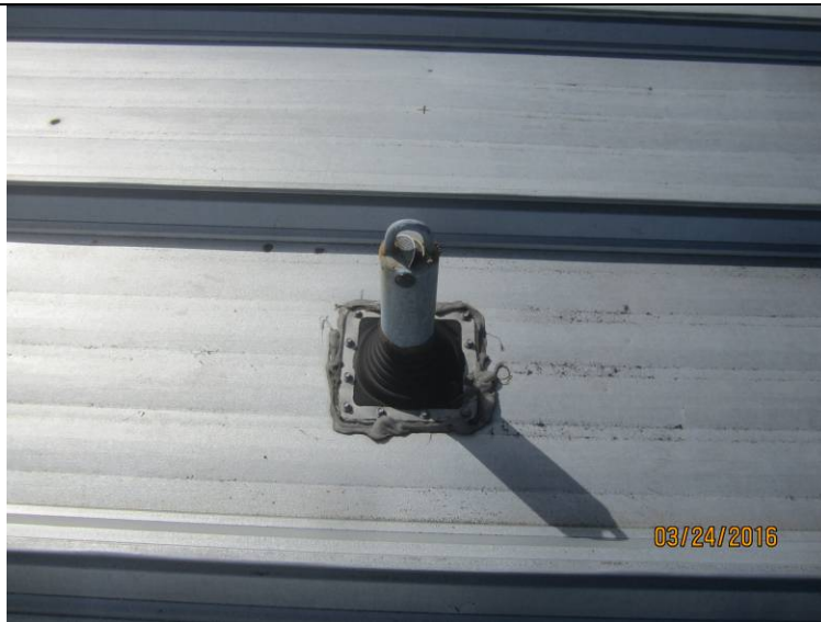
Photograph 13: Sealant applied at the transition between the through roof penetration flashing and the metal roof panel.
