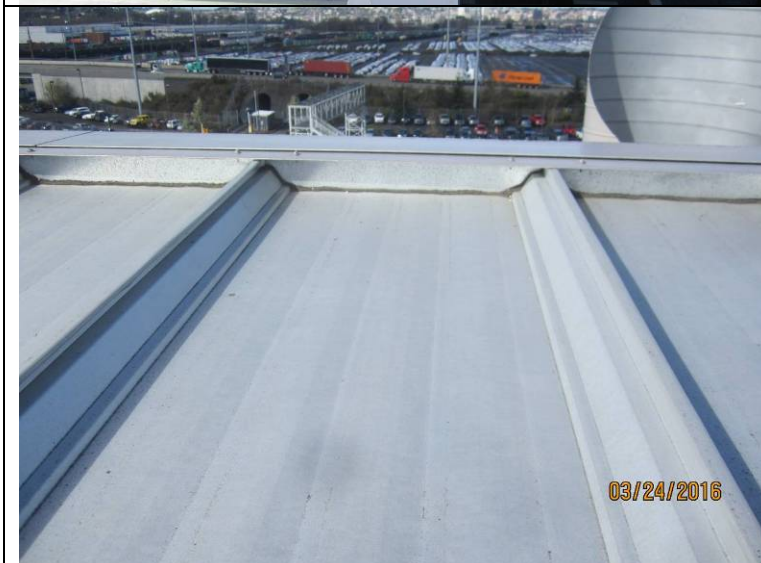
Photograph 6: Looking upslope at the upslope edge flashing and z-closure.
