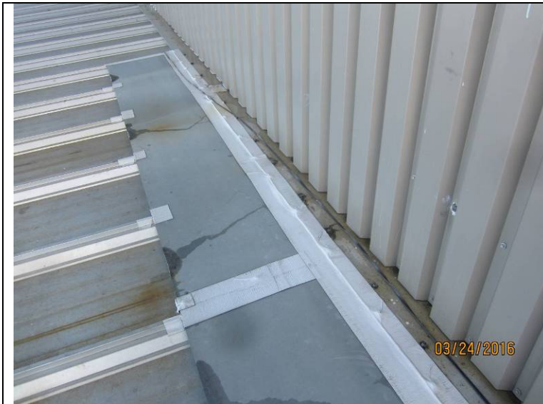
Photograph 22: EternaBond tape applied at the added flashing laps and transition to the existing flashing.
