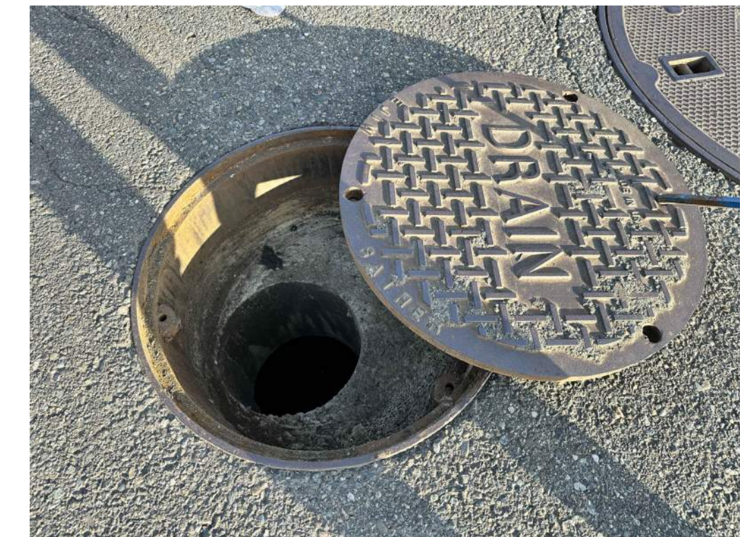
4 PHOTO - EX DETENTION VAULT
