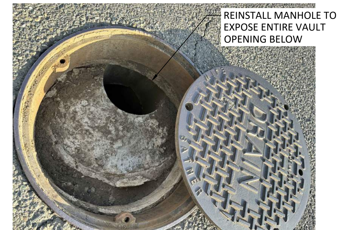
5 PHOTO - EX DETENTION VAULT
