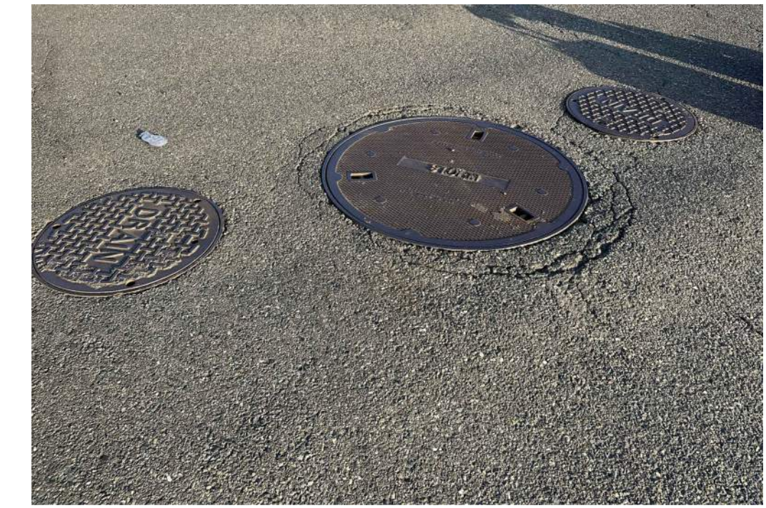
3 PHOTO - EX DETENTION VAULT
