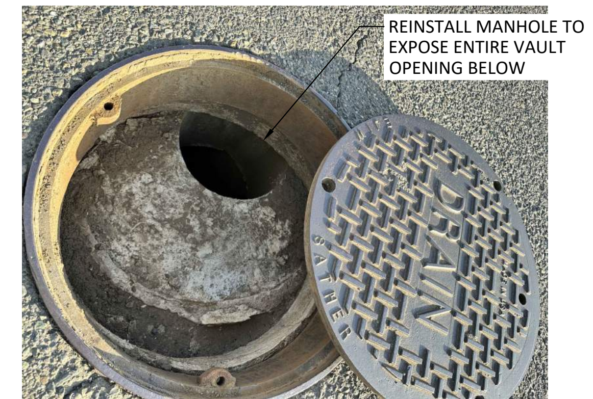
5 PHOTO - EX DETENTION VAULT
