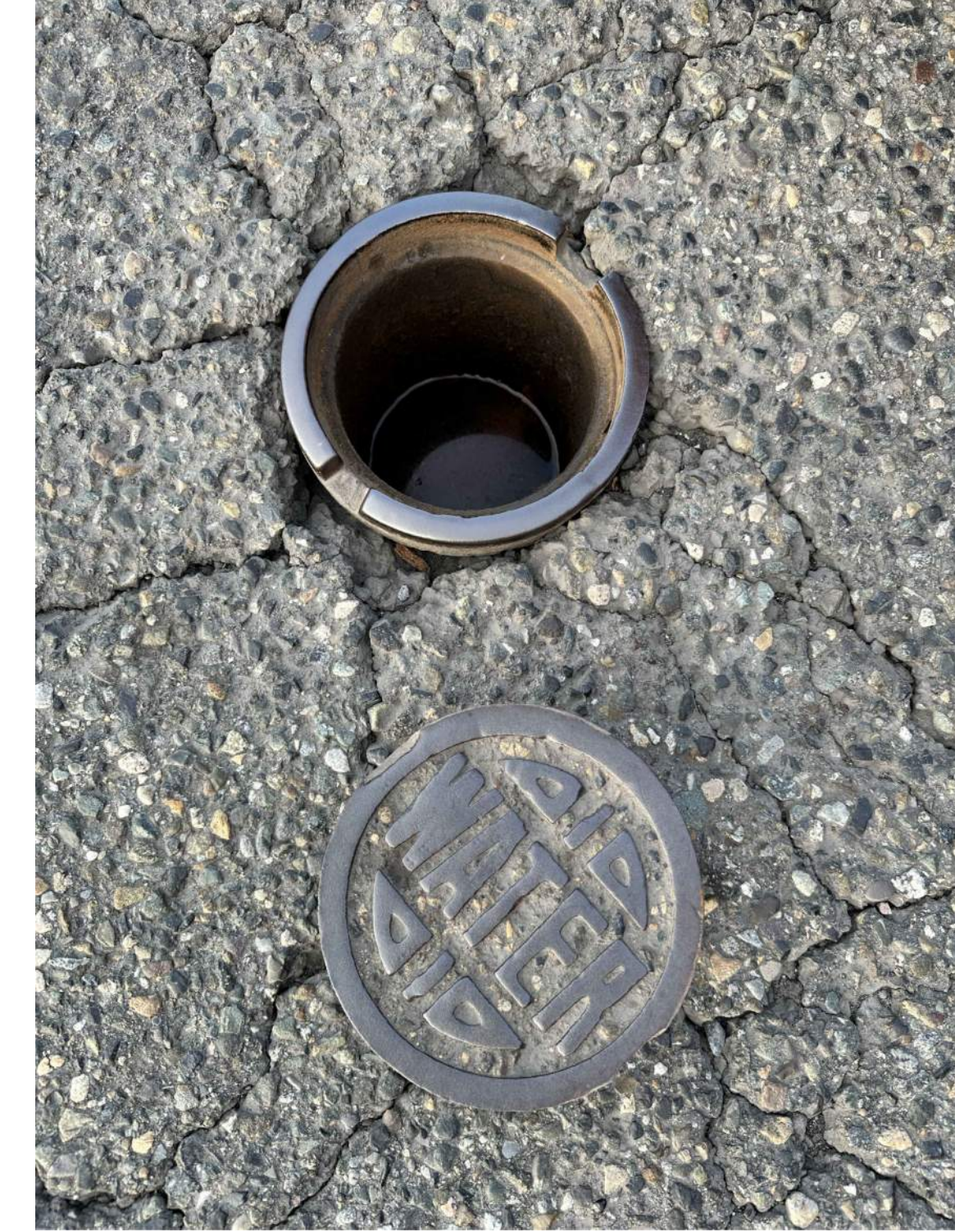
5 PHOTO - TYP EX WATER VALVE
