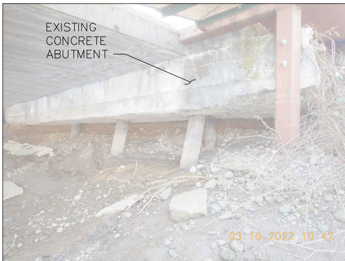
EXISTING CONDITIONS SCALE: NTS
