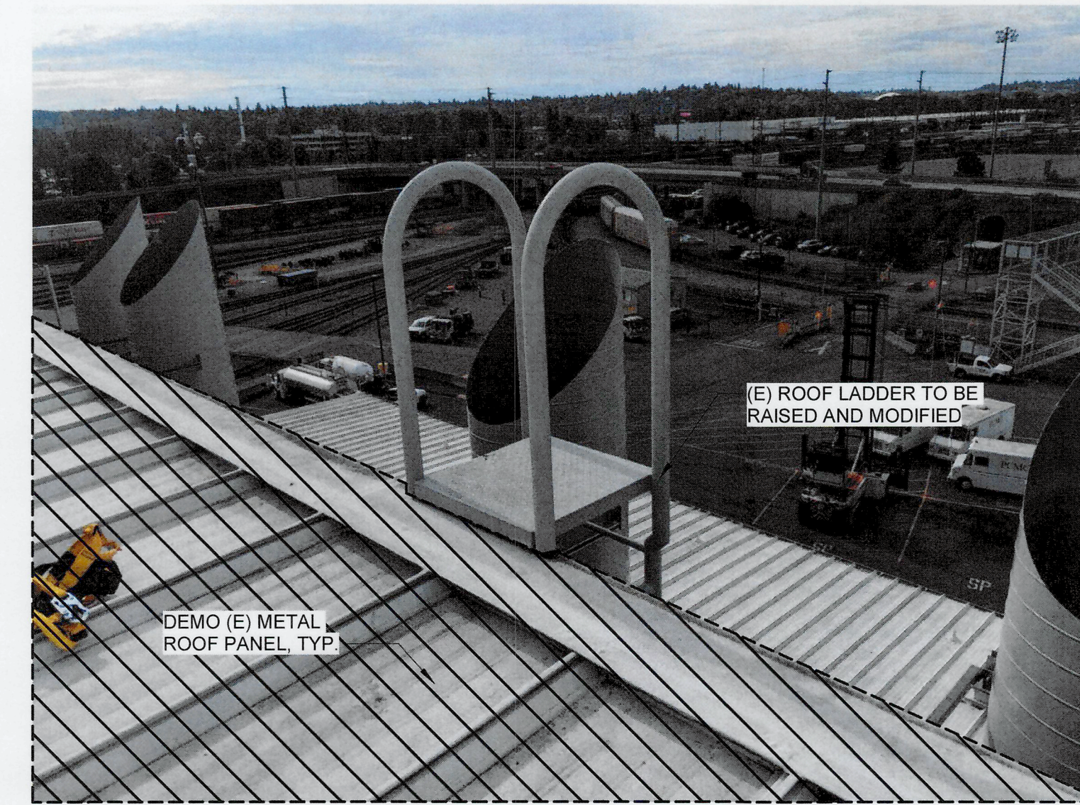
3 (E) ROOF ACCESS LADDER NTS
