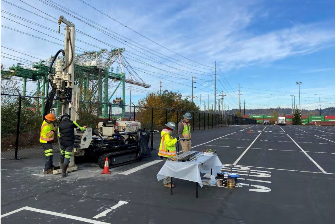
Figure 8. Boring for AB-2 with direct push drill, view northwest.
