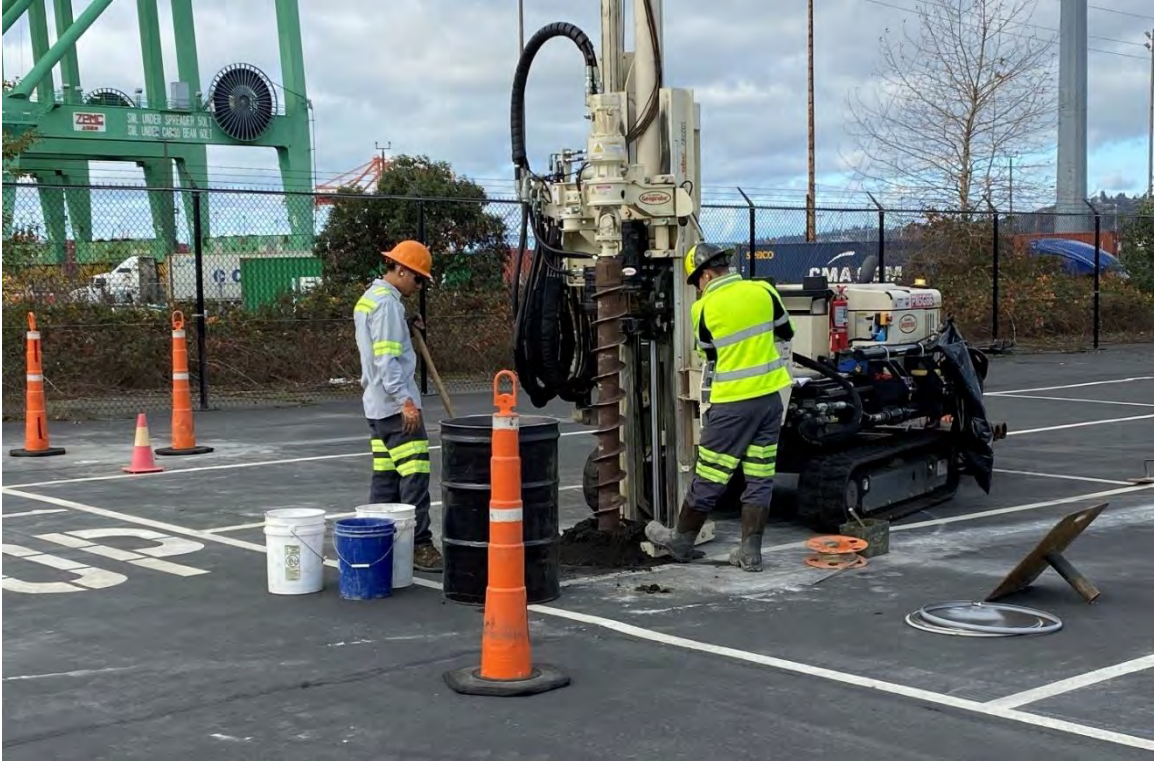
Figure 7. Drilling MW-14 with 6” auger and shoveling spoils for inspection. View northwest.
