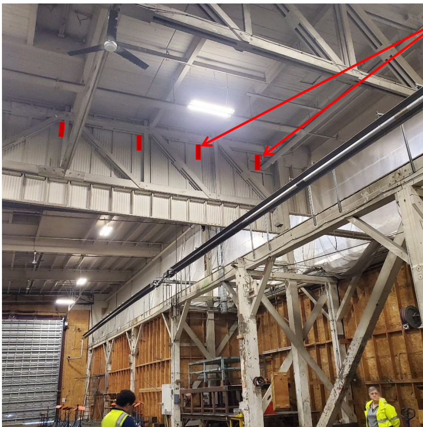
Photo 4: Existing Draft Curtain at Gridline G
