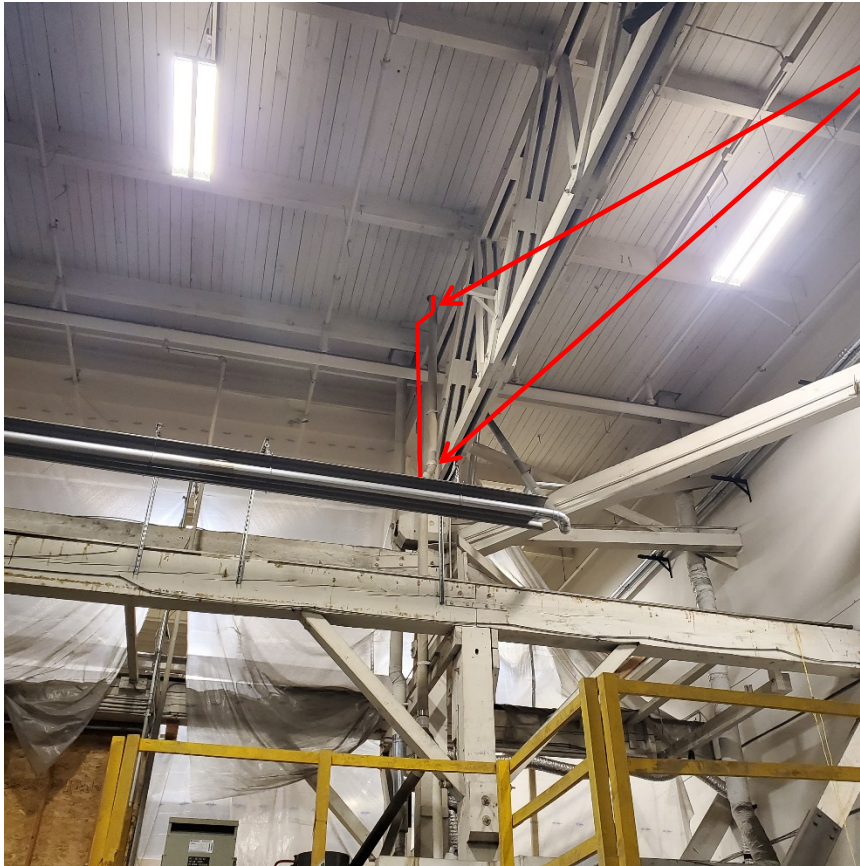
Photo 3: Existing Rainleader at Grid E-13
