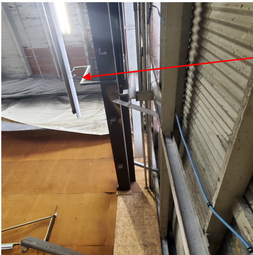
Photo 6: Radiant Tube Support Modifications
