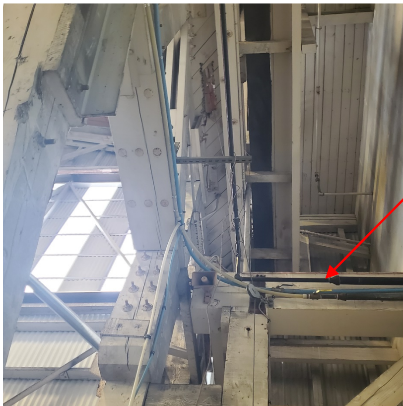
Photo 2: New Gas Piping Shut-Off Valve
